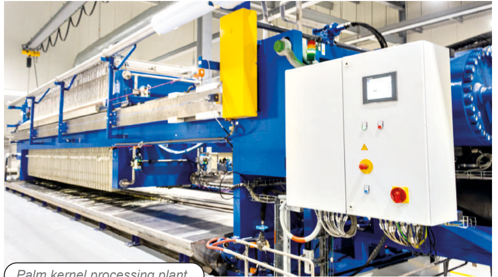
Palm kernel processing plant
